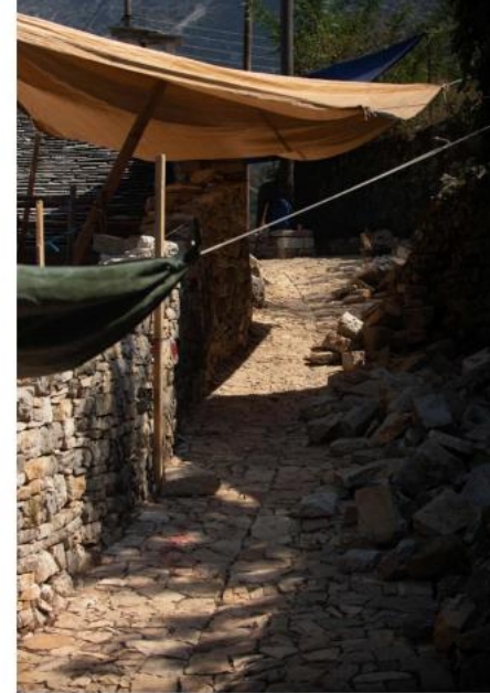
Works in progress (11)
