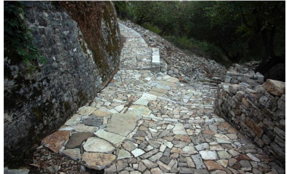
Part of the restored cobble pathway (17)
