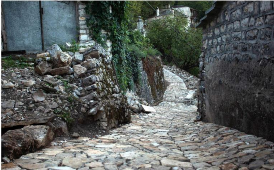
Part of the restored cobble pathway (18)
