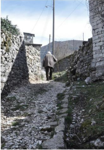
The dilapidated kalderimi of Aristi. Condition on site (03)
