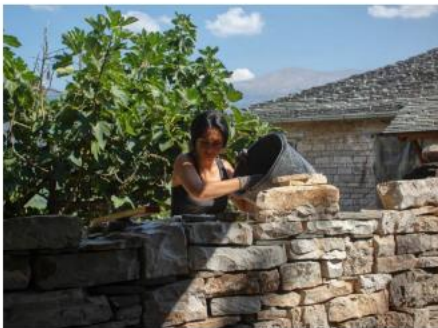
A participant working on the dry-stone retaining wall (09)
