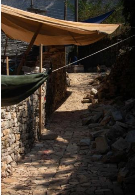
Works in progress (11)
